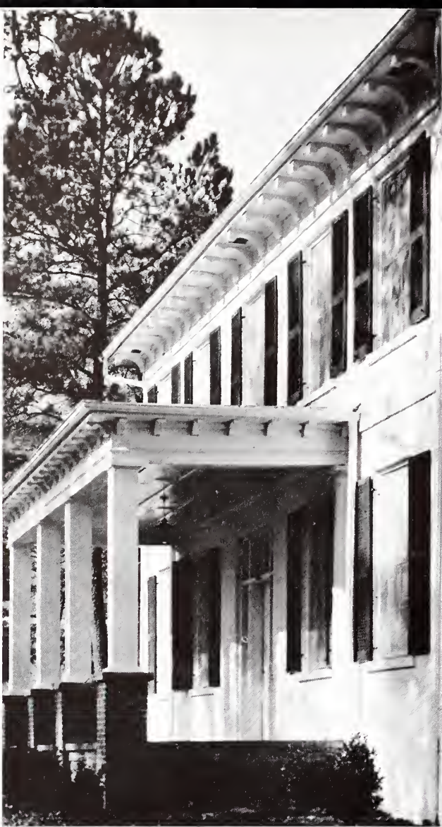
STUDENT PERSONNEL BUILDING
